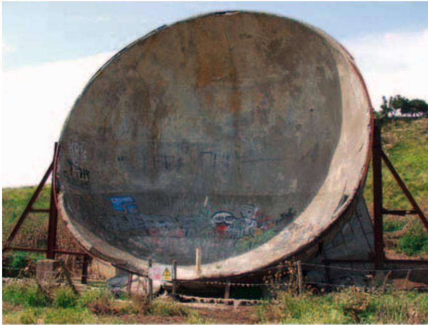
Prior to World War II and the invention of radar, concrete *Acoustic Mirrors* were built to reflect sound waves as early warning devices around the coasts of Great Britain
